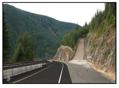
Project includes placing about 2.5 miles of center barrier to prevent crossover crashes. A gap is provided for emergency use only at the runaway truck ramp.
